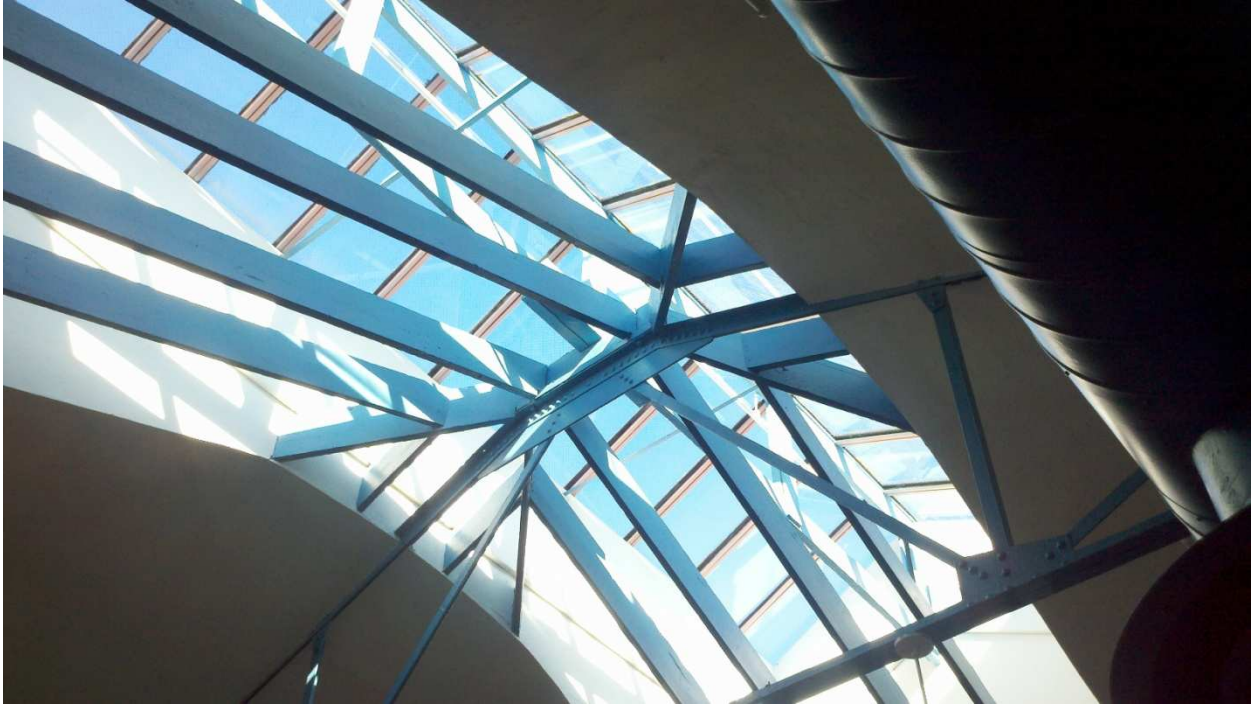
Photograph 2 – Roof framing in the central atrium of Trinkle Hall. In this photograph the primary roof supporting element is a steel truss, while the secondary framing consists of wood joists.
