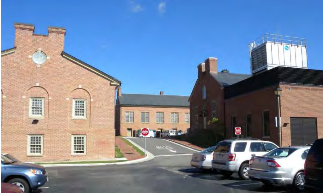
Facilities Management (l) and Main Power Plant (r) with Trinkle in background
