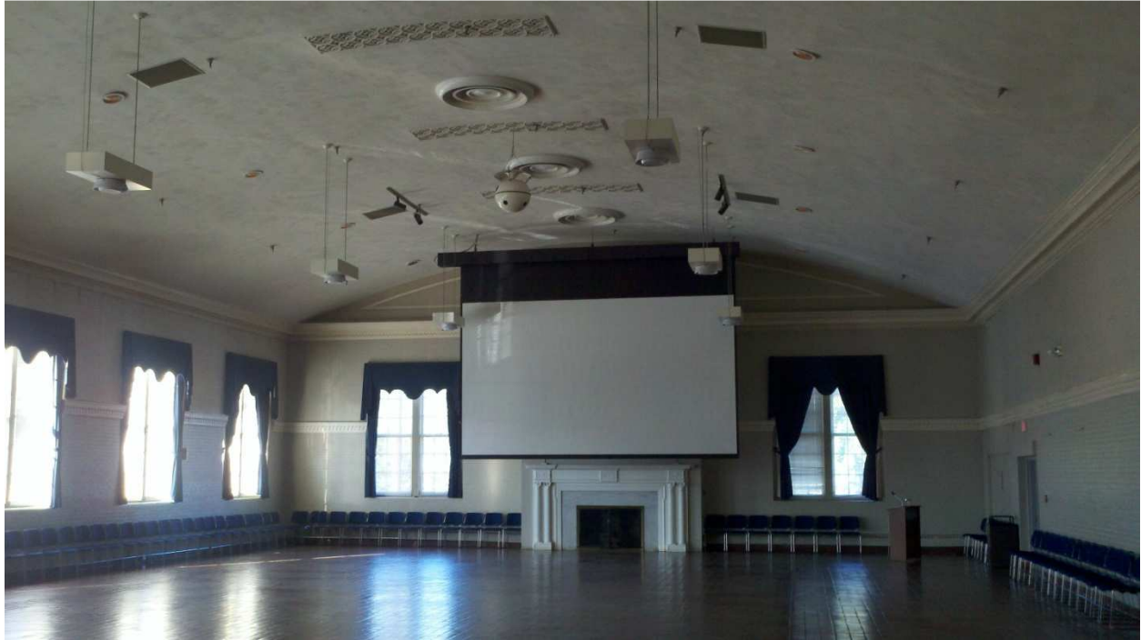
Photograph 1 - Large volume space that was originally used as a dining hall. The primary members of the roof framing consist of steel peaked trusses with a curved bottom chord and we anticipate the secondary framing consists of wood joists and decking.
