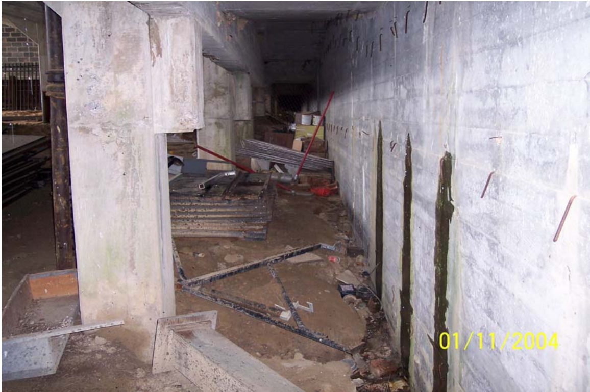
Photograph No. 27 Typical soil erosion at inner wall
