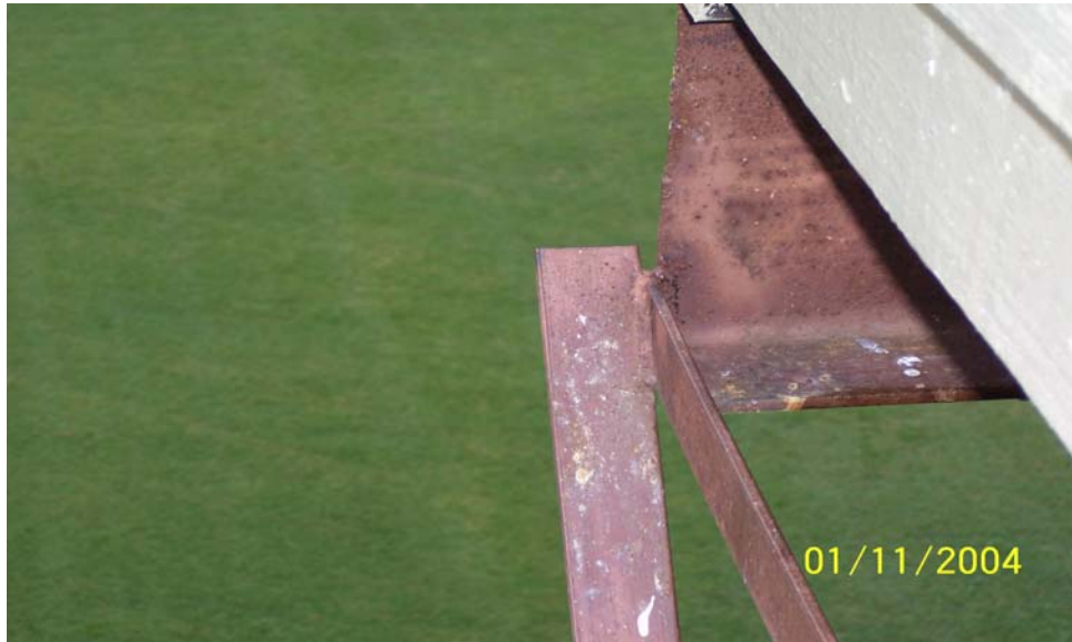
Photograph No. 9 Typical connection at knee brace consists of tack welds to 2 inch flatbar
