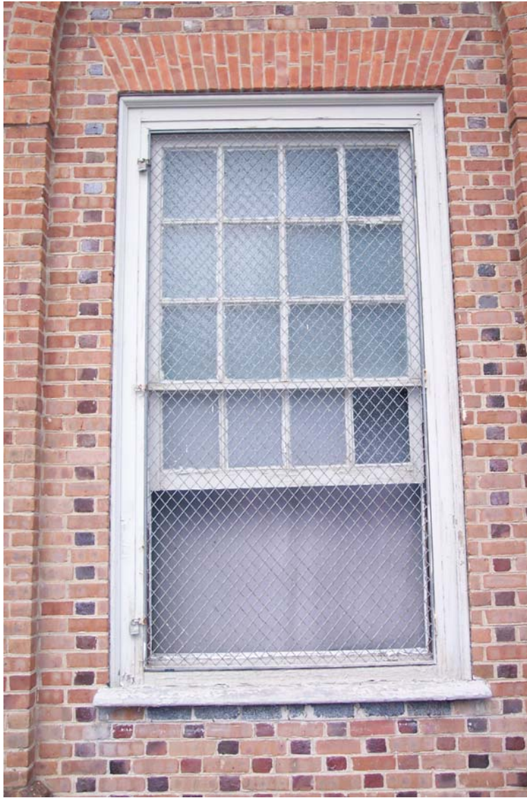
Photograph No. 1 Typical paint scale chipping at windows
