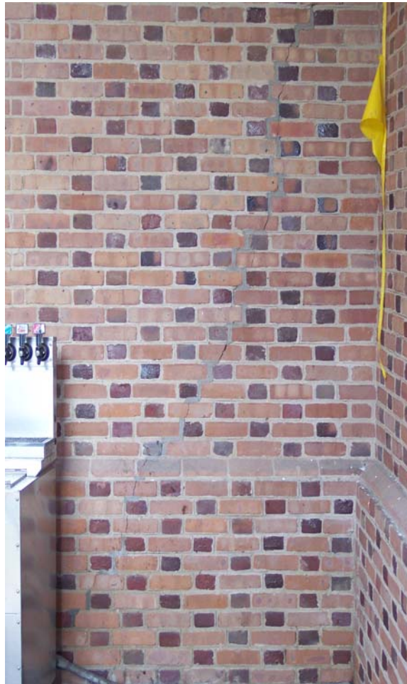
Photograph No. 3 Vertical crack propagates through the brick and mortar joints. This crack goes completely through the wall. SW corner of Pavilion No. 6
