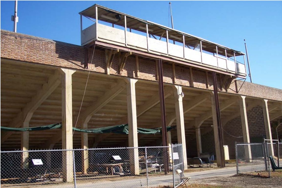
Photograph No. 7 Steel shoring on wooden press box.
