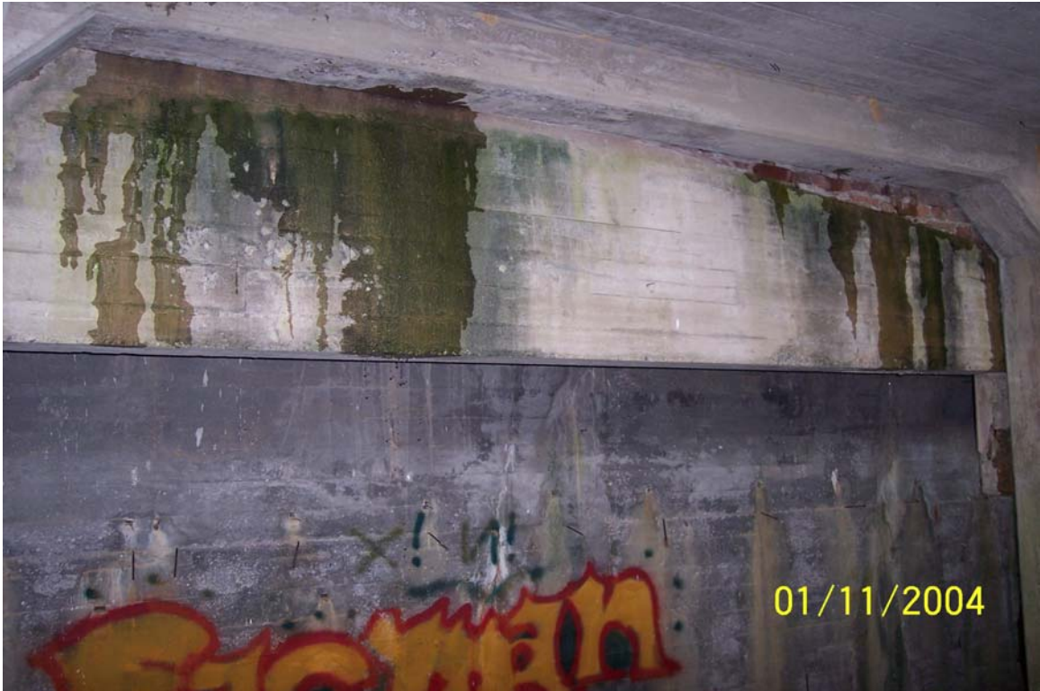
Photograph No. 25 Leaking joint at lower brick wall and supporting concrete beam
