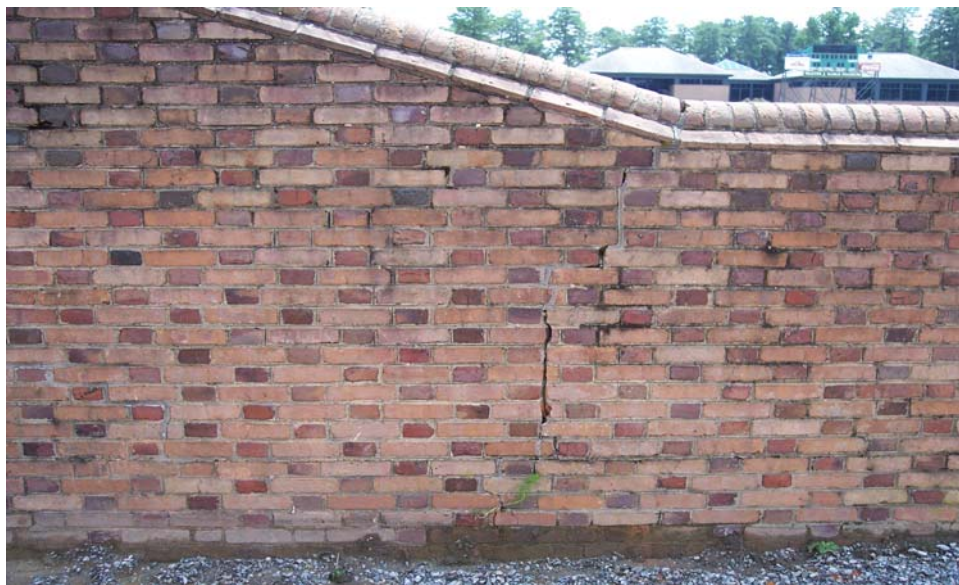
Photograph No. 10 Typical foundation settlement crack on all four brick wingwalls. Underside of deck has erosion due to water infiltration from clogged floor drains
