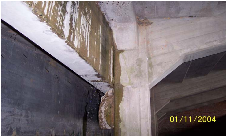
Photograph No. 20 Leaking joint where lower inner wall abuts deck. The transfer beam spanning between the frames supports the inner brick wall. Notice severe spalling of corbel due to water.
