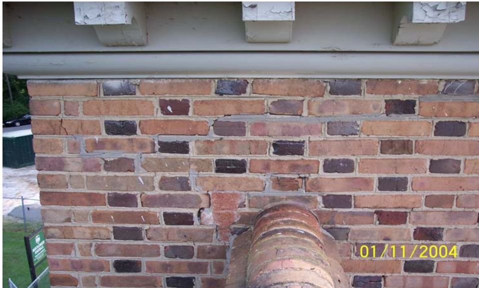
Photograph No. 17 Thermal expansion of upper walls have “punched” through the wall at Pavilion No. 6
