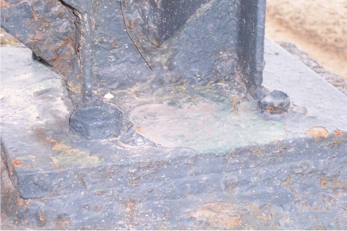
Photograph No. 9 Missing anchor bolt at stadium sign base plate. Also notice the rusting at the bracing connections
