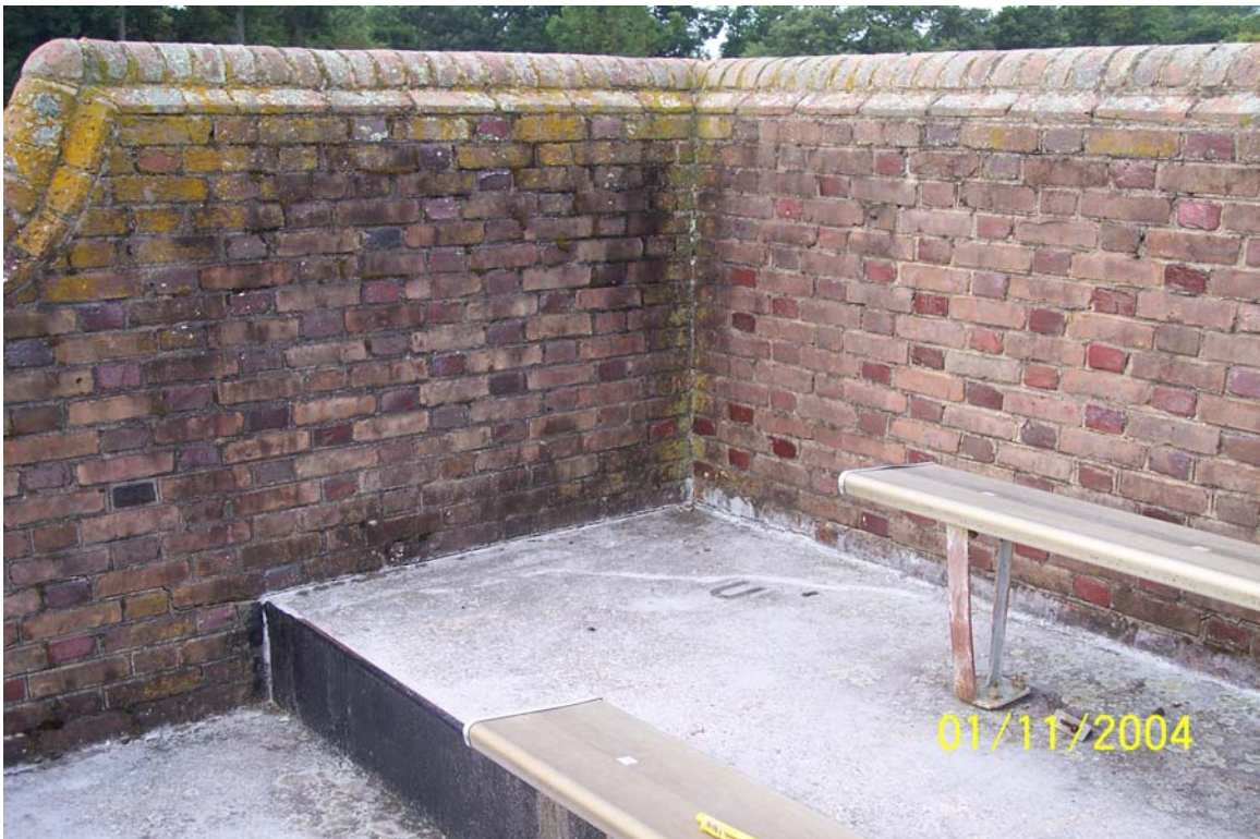
Photograph No. 4 Full view of wall cracks at southwest corner of stadium. Cracks extend up from deck to top of wall and follow temperature crack in deck
