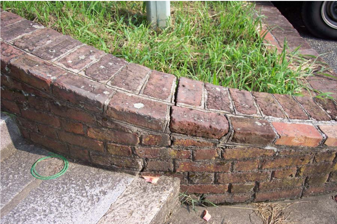
Photograph No. 8 Crack in stair retaining wall
