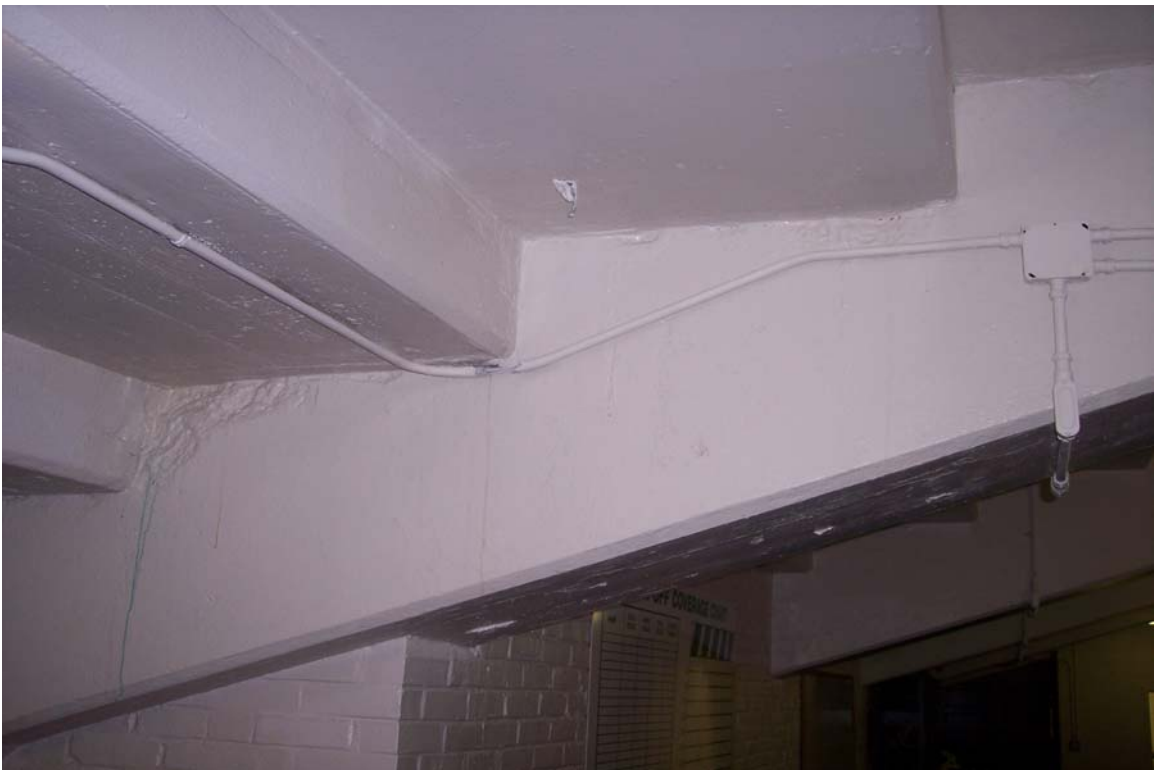
Photograph No. 20 Interior bearing spalls along top of concrete frame at column line 17 inside the locker room. Notice no water stains are present
