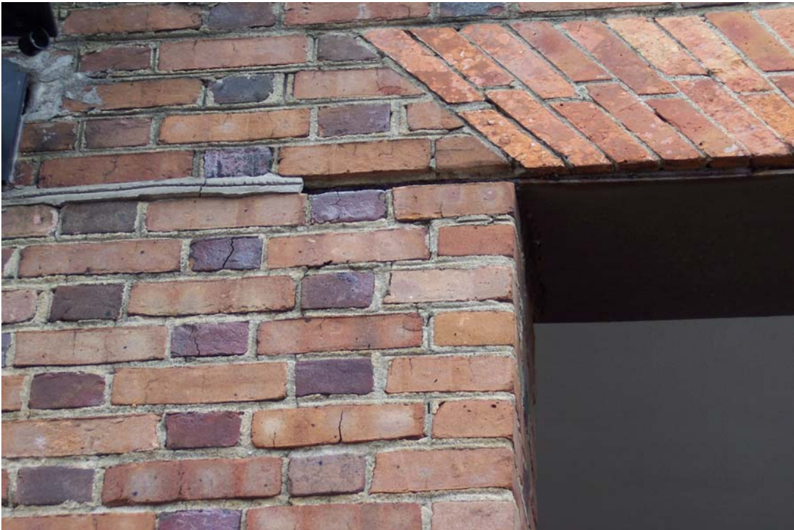
Photograph No. 14 Rusted shelf angle. Notice expansion of steel due to erosion has broken out previously repaired mortar joint
