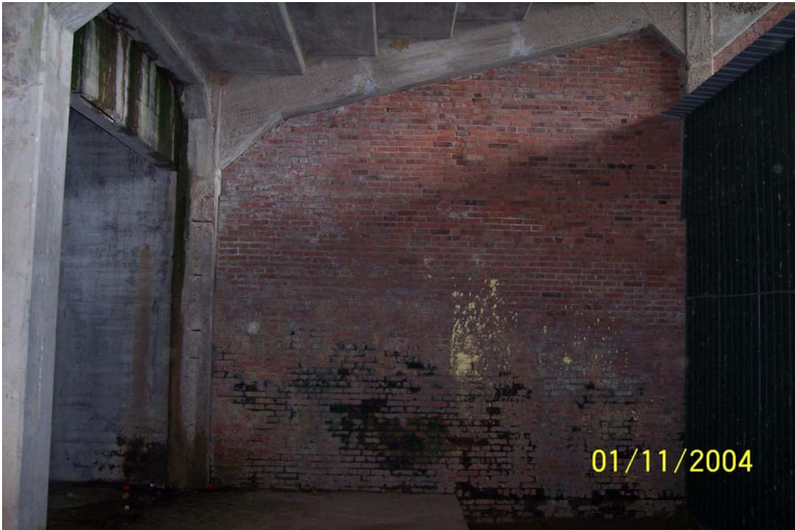
Photograph No. 28 Brick wall at south end of stadium. This wall supports the outside stairs as seen in Photograph No. 6 in the Arcade, Pavilion Photograph section
