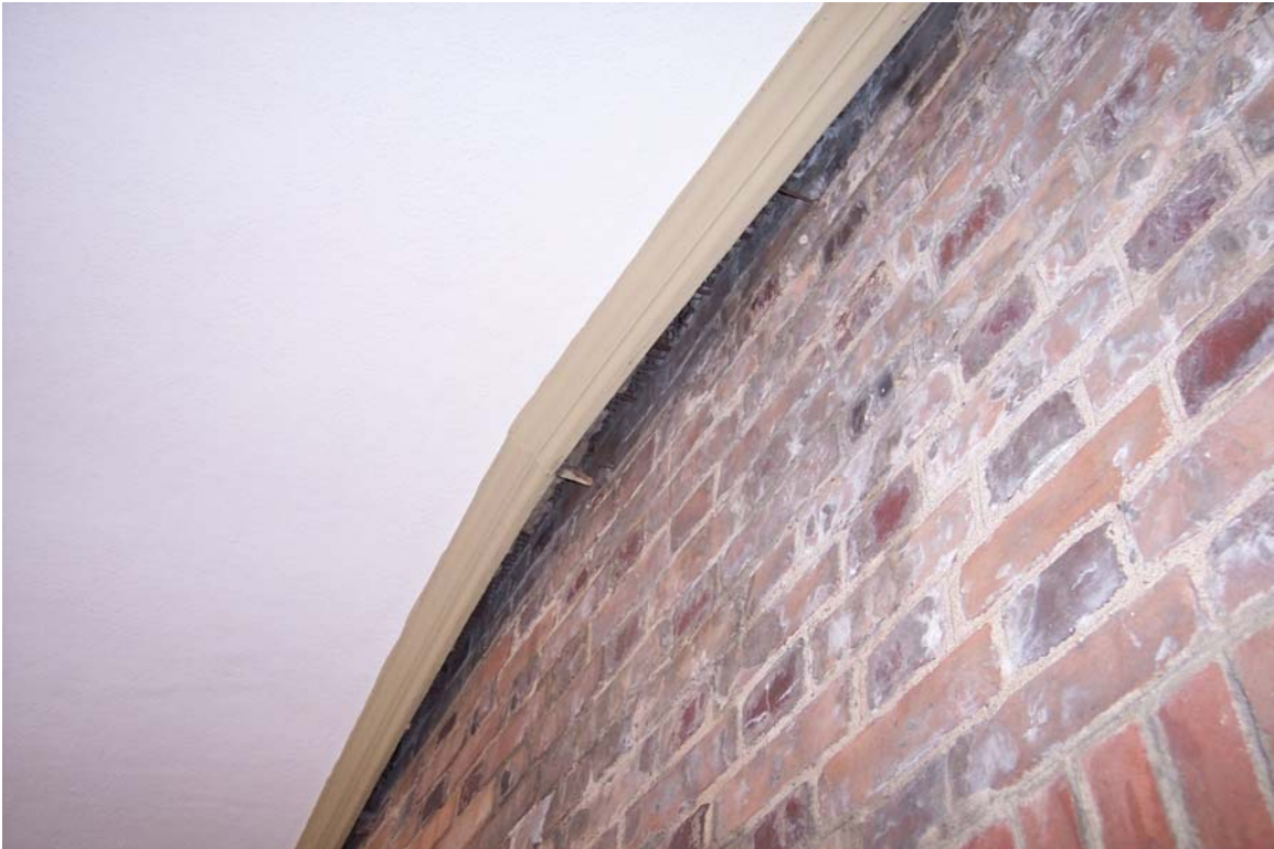
Photograph No. 17 Wood nailers have pulled out of brick. The wood trim could pose a safety hazard should it fall.
