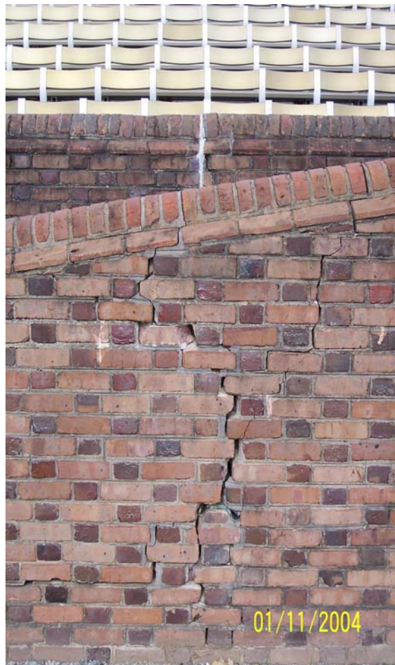
Photograph No. 14 Large crack and brick movement in lower walls at column line 19 due to thermal expansion at construction joint
