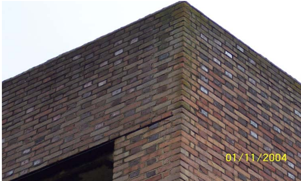
Photograph No. 5 Crack at southwest corner. Notice brick has moved away opening at a result of thermal expansion
