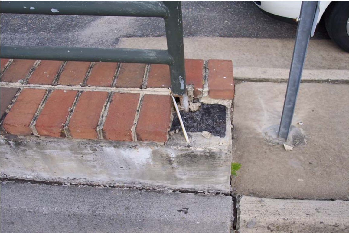
Photograph No. 5 Same retaining wall. Missing brick
