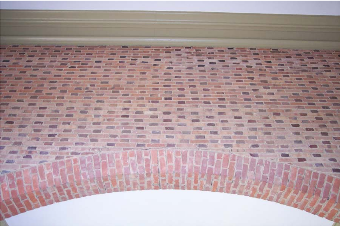
Photograph No. 1 Typical vertical crack at brick keystone
