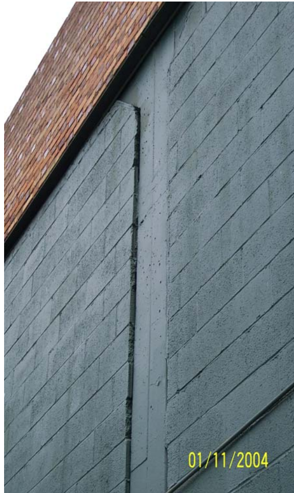
Photograph No. 19 CMU infill wall at column line 22 has tilted outward from frame
