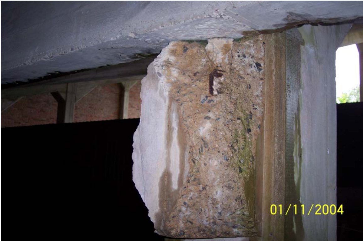
Photograph No. 21 Extensive spalling at concrete corbel
