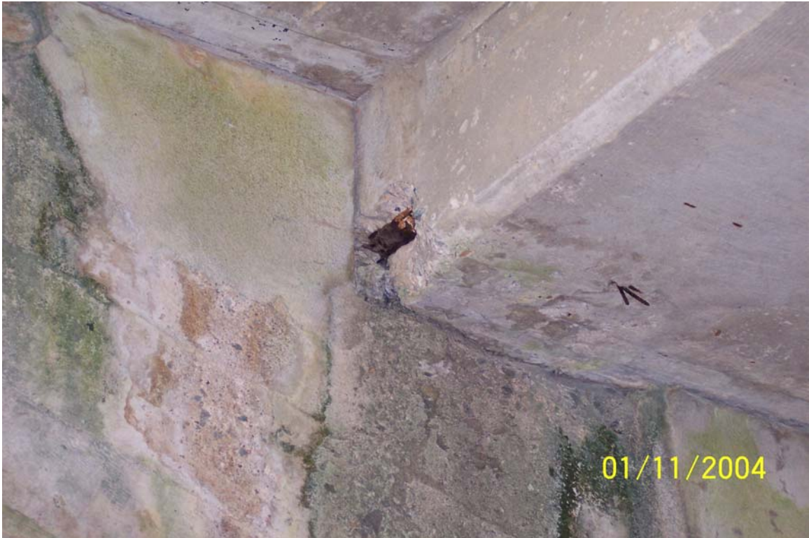
Photograph No. 23 Close up of spalling at bearing seats. Notice exposed main reinforcement due to lack of concrete cover
