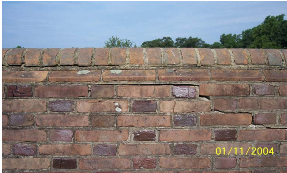
Photograph No. 13 Enlarged photo of crack in upper wall at column line 19 construction joint
