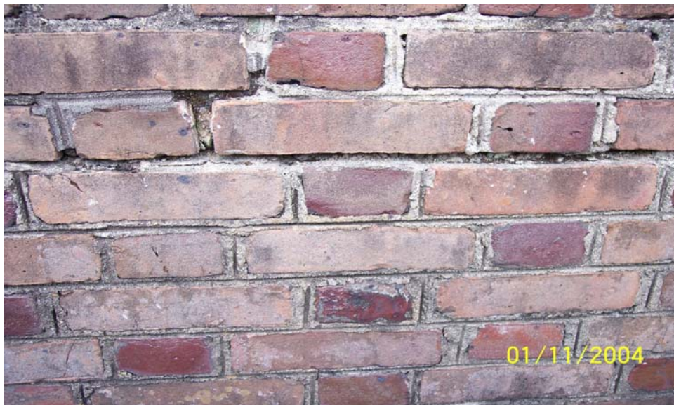
Photograph No. 16 Typical brick mortar joints requiring re-pointing
