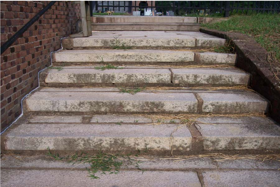
Photograph No. 6 Stairs at south end of West Stadium have cracks or opened joints. Notice the wall to the left is acting as a retaining wall to the open pit below
