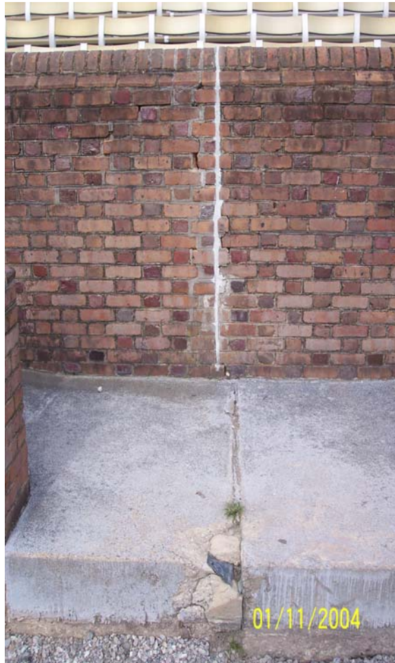
Photograph No. 15 Crack in lower walls at column line 13 due to thermal expansion at construction joint. Past crack was repaired
