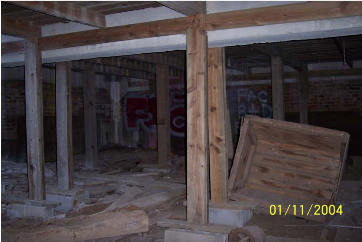
Photograph No. 29 Timber framing supporting the maintenance area
