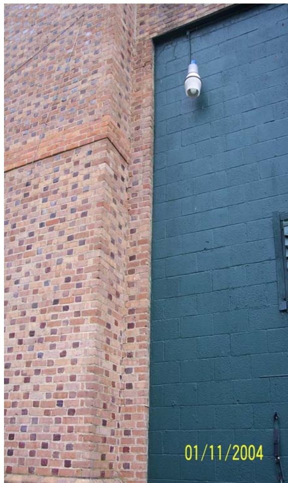
Photograph No. 18 The thermal expansion shown in Photograph 17 has created a full height vertical crack at the wall intersections
