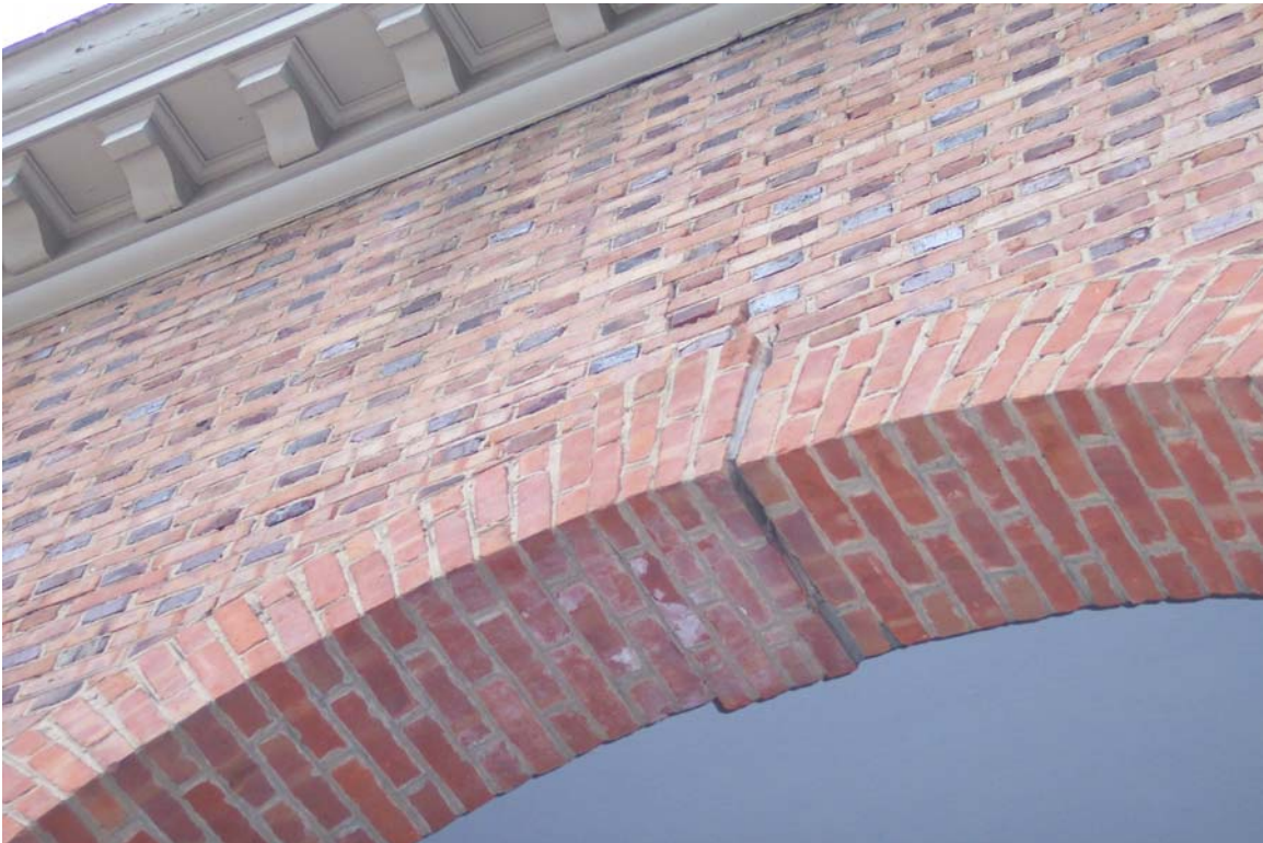
Photograph No. 6 Vertical crack at brick key in arch. The key has dropped down. Crack continues up vertically to the soffit
