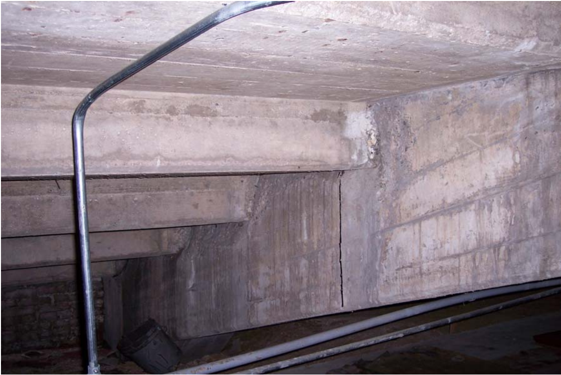
Photograph No. 19 Bearing spalls along top of concrete frame at column line 17
