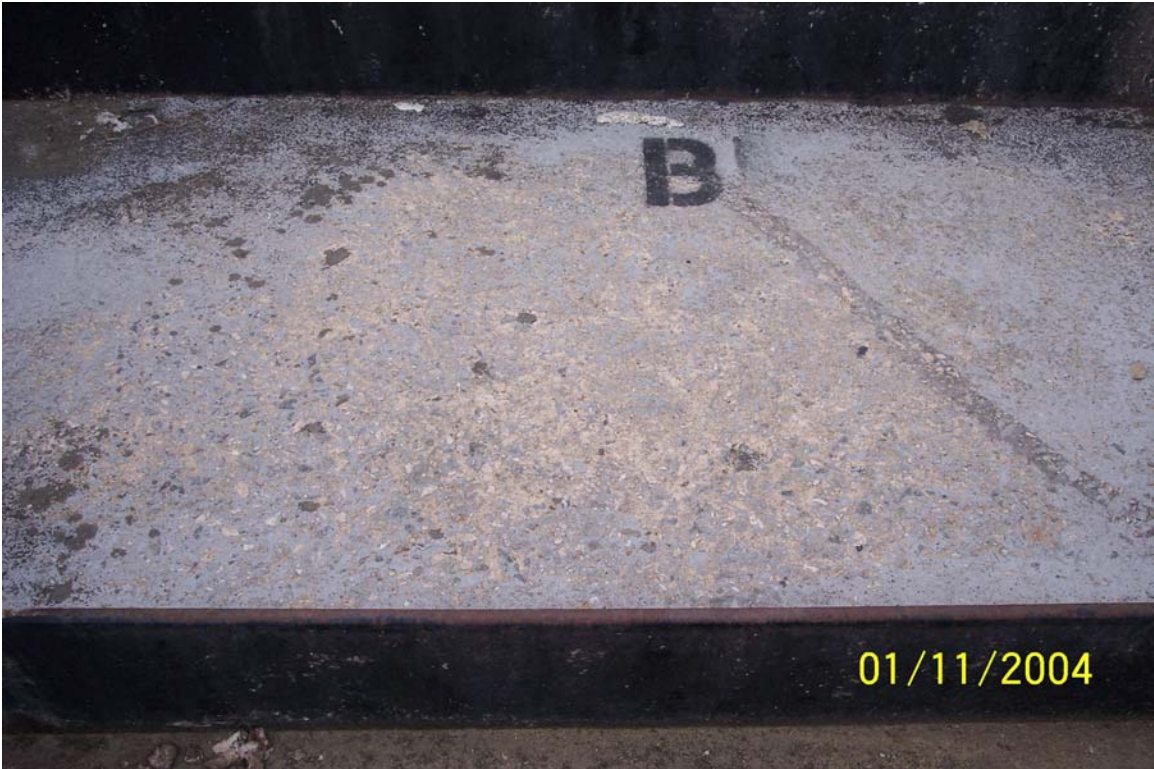
Photograph No. 1 Typical Light Abrasion to Concrete Deck and wear to the coating system
