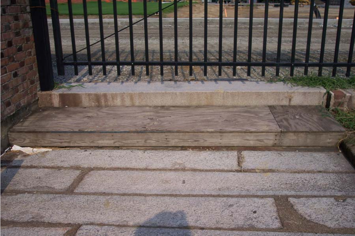
Photograph No. 7 Additional wood step installed to reduce riser height. No signs of settlement were present
