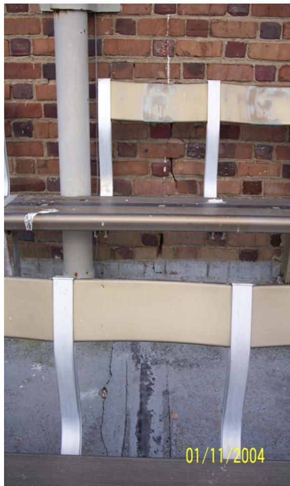
Photograph No. 10 Crack in inside of upper wall and spall in construction joint at column line 13
