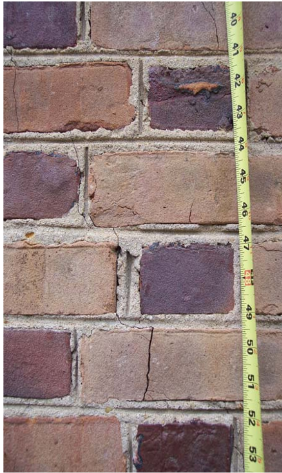
Photograph No.3 Cracks extend through the bricks and follow the mortar joints
