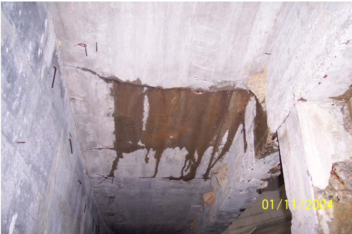
Photograph No. 24 Transverse temperature cracks leaking. This is the concrete ramp between the two lower walls.
