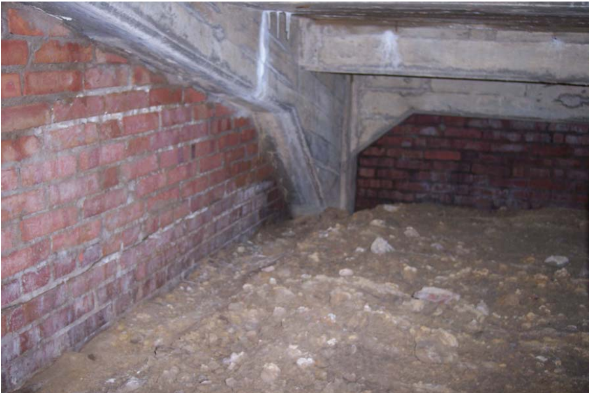
Photograph No. 12 Typical erosion/washout of interior wingwall
