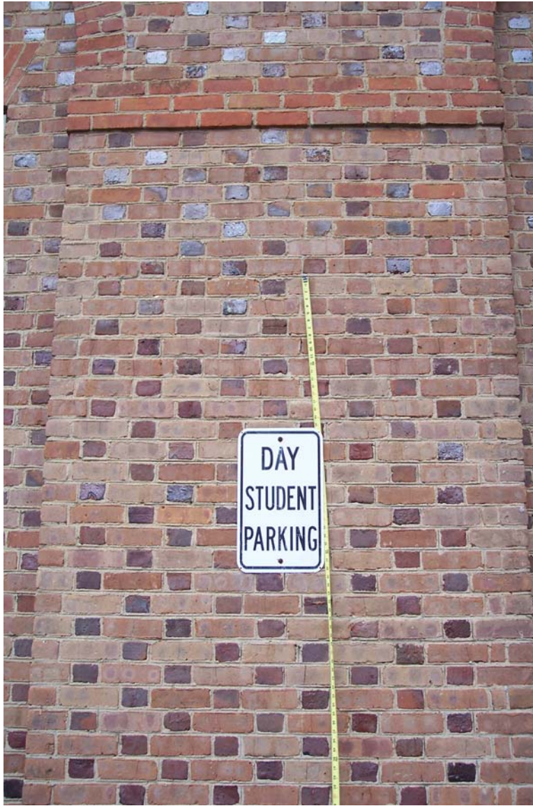
Photograph No. 2 Hairline vertical crack in brick mortar joints and through bricks
