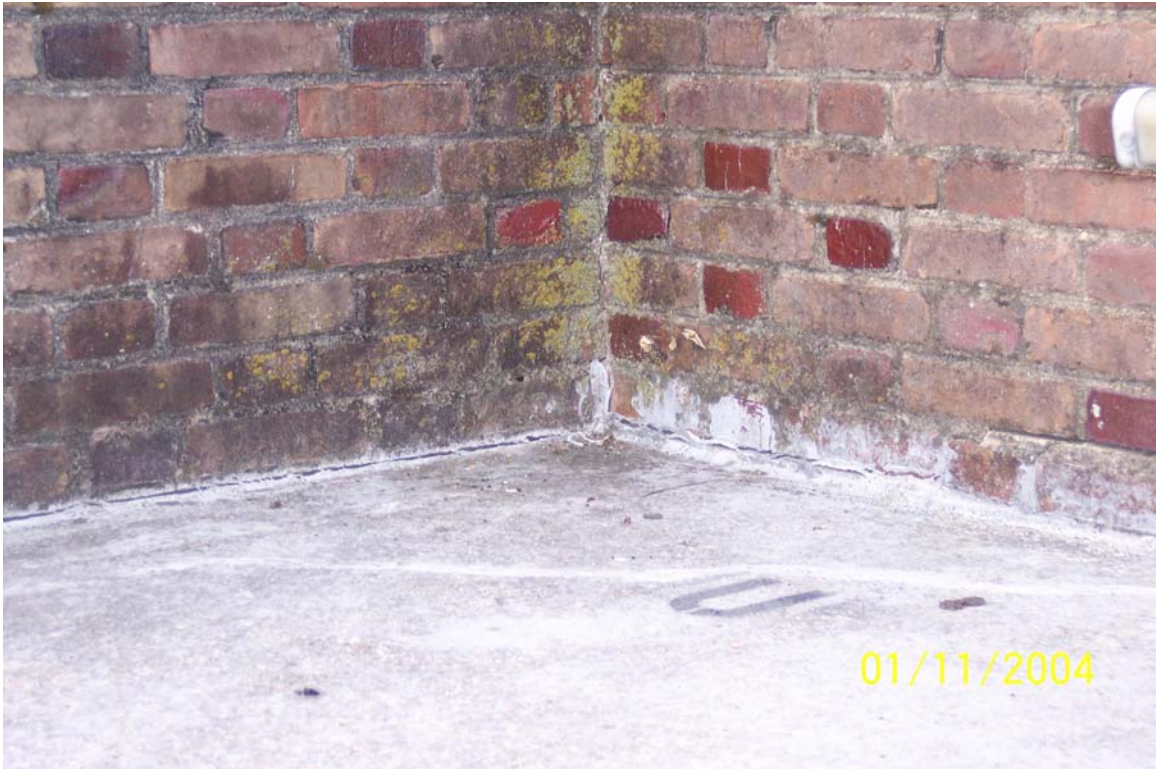
Photograph No. 3 Horizontal crack at base of concrete deck. Notice temperature crack diagonal to wall corner.
