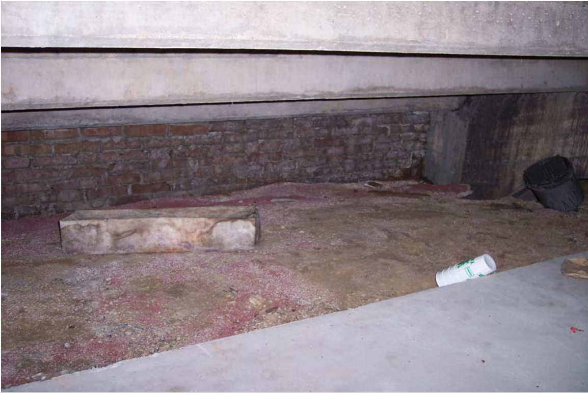
Photograph No. 11 Washout and erosion under at lower wall directly under floor drains
