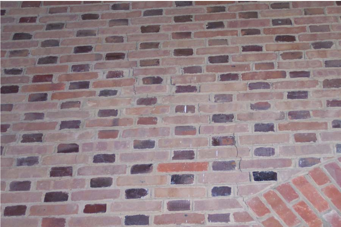
Photograph No. 2 Typical stairstep mortar joint crack at bottom of brick arch
