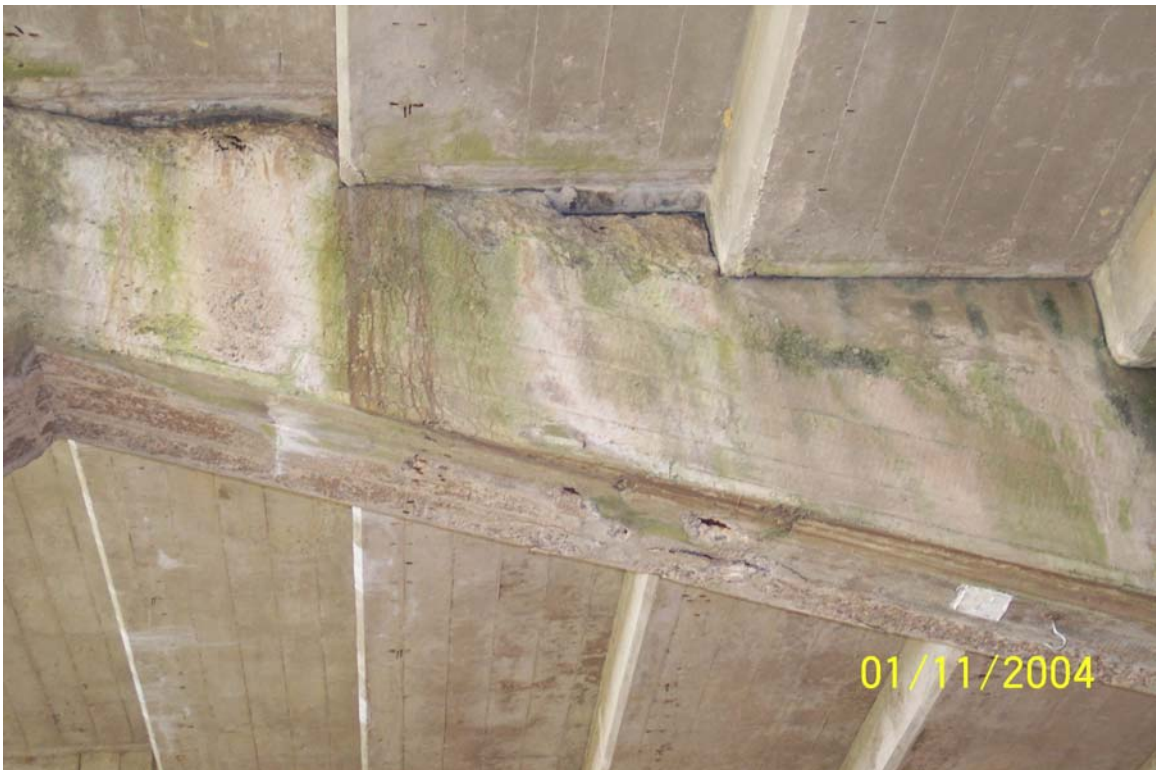
Photograph No. 22 Concrete spalling of bearing seats at construction joints at column lines 7, 14 and 19.
