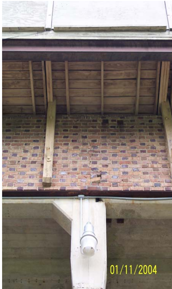
Photograph No. 11 Crack on outside of wall at column line 13. Notice loose brick just above light fixture.
