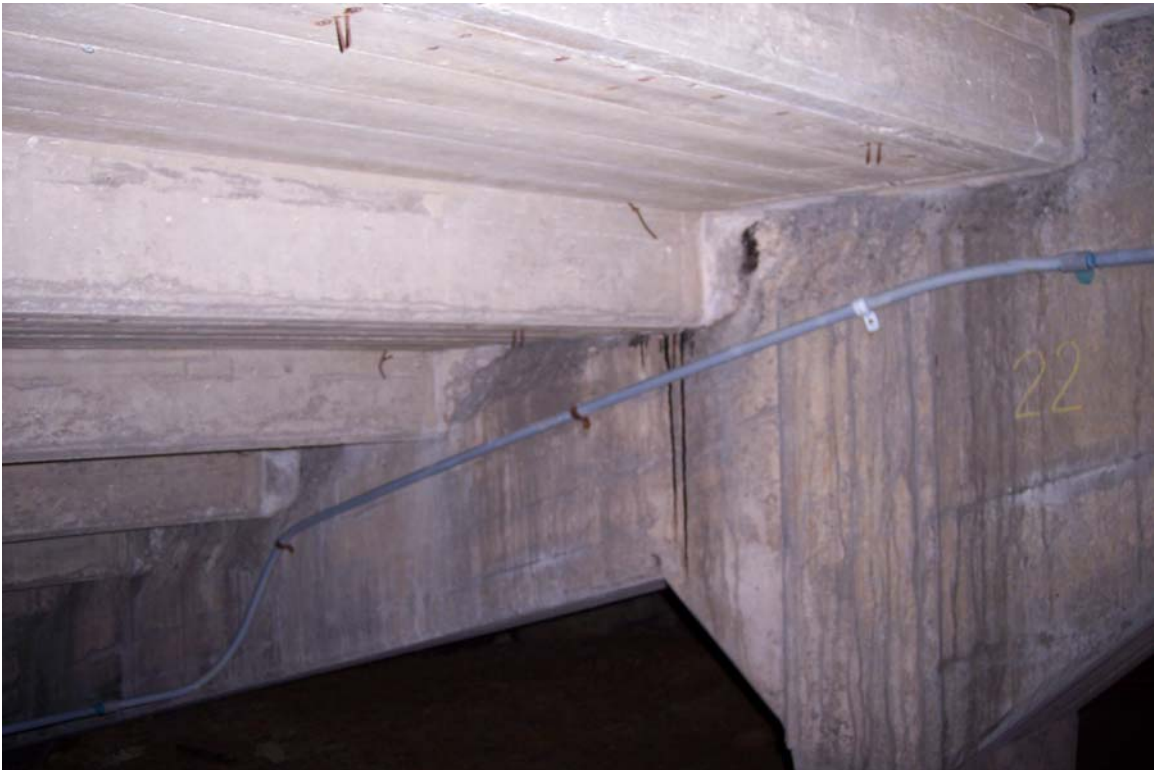
Photograph No. 18 Bearing spalls along top of concrete frame at column line 22
