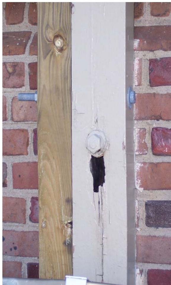
Photograph No. 6 Typical extensive wood rot on press box posts (Note: 4x4 posts added later for strengthening)
