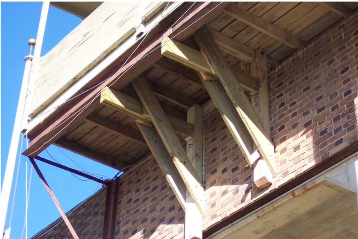
Photograph No. 8 Typical knee brace at each end of press box shoring (Note: wood knee bracing added later for strengthening)
