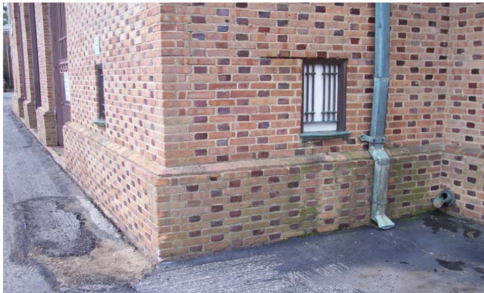
Photograph No. 4 Full view of vertical wall crack at the ticket office along column line 15. Notice presence of ponding water adjacent wall at crack. These are in close vicinity of the roof drain and rain water leader. This is typical on the opposite side
