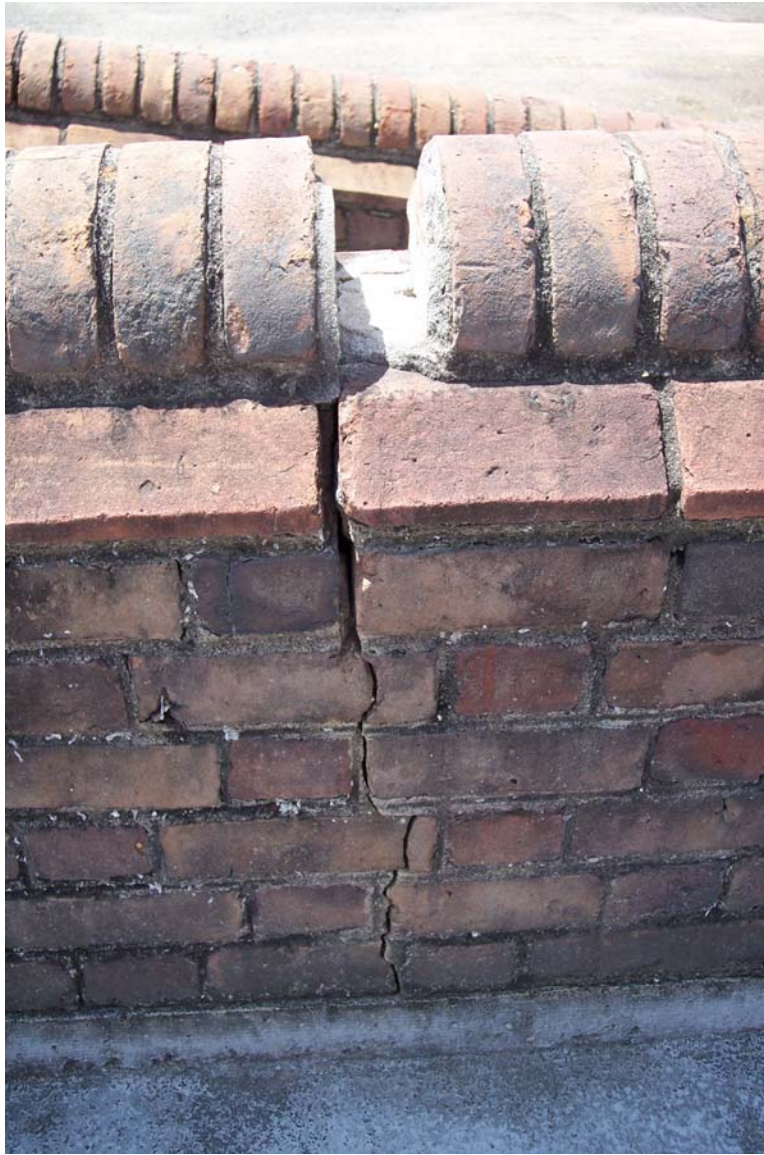
Photograph No. 8 Large thermal crack in lower brick wall
