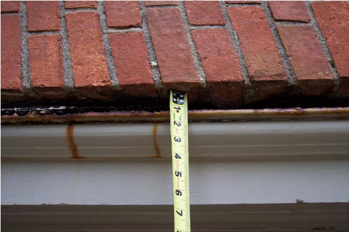
Photograph No. 13 Severely rusted shelf angle
