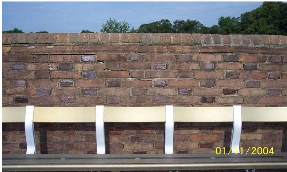
Photograph No. 12 Crack in upper inside wall at column line 19 construction joint
