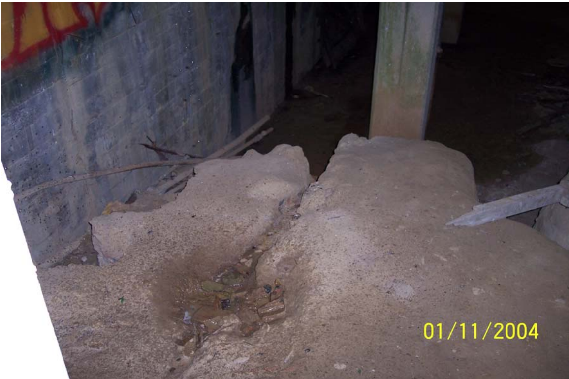
Photograph No. 26 Soil erosion at inner concrete wall which support outer brick wall
