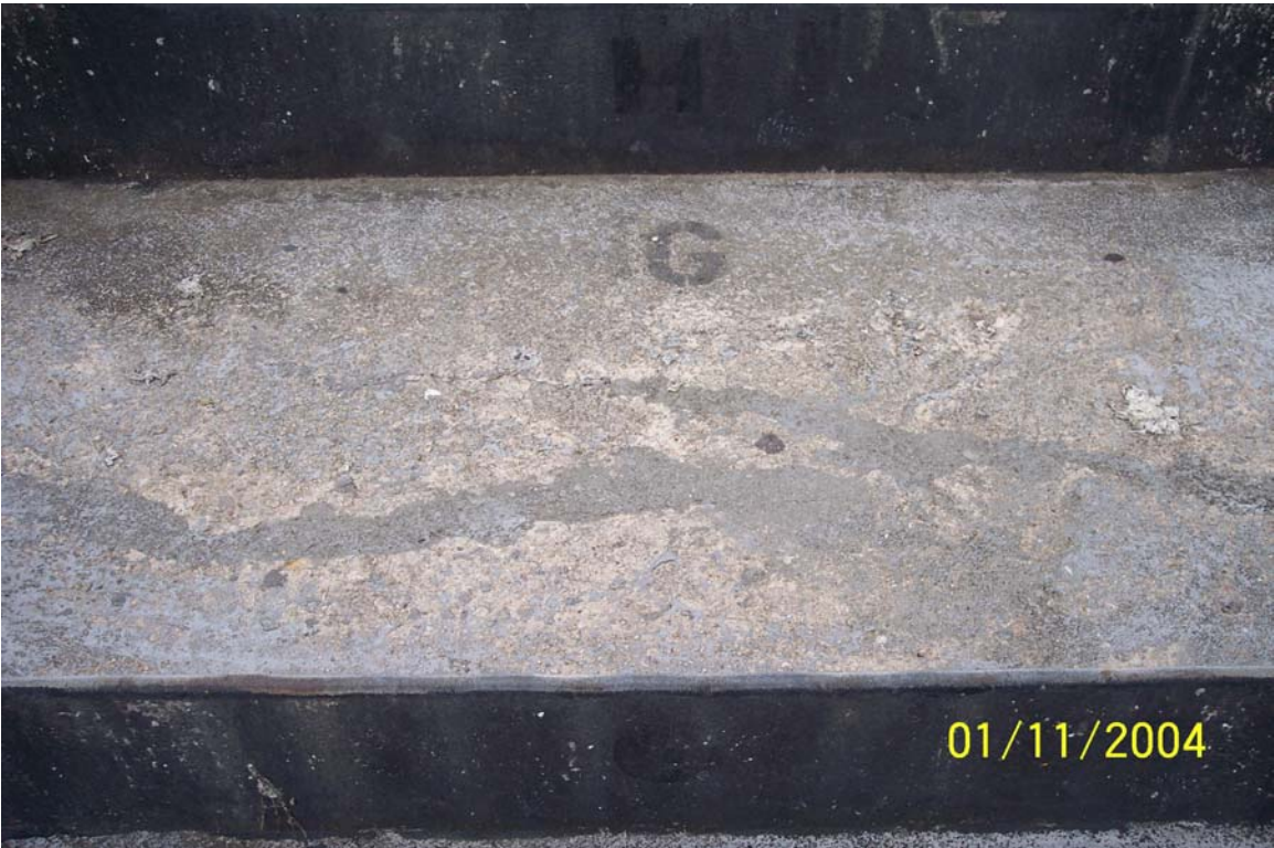
Photograph No. 2 Typical Moderate Abrasion to Concrete Deck requiring chipping away of loose aggregate
