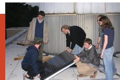
Mounting of the 176-watt panel on its rack, just after Spring Break.
